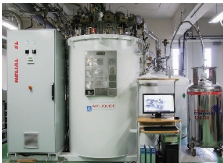
Fig. 1: Helium liquefier in CL
